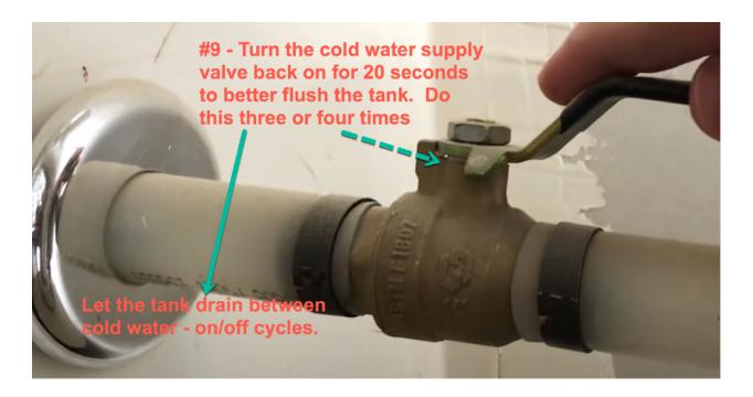
The video recommends filling the tank completely, then draining it one more time.
